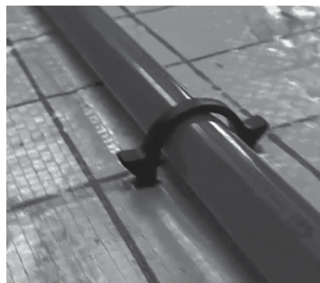
Ensure that the clips are fixed securely
