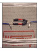
12 Slide one small piece of heat shrink over both sections of exposed earth braid. Cut a section of the "bridge" wire provided to a length suitable to replace the wire removed from the heating element. Strip 10 mm from either end of this wire into the butt crimps located on the ends of the earth braid and crimp using the crimping tool.
